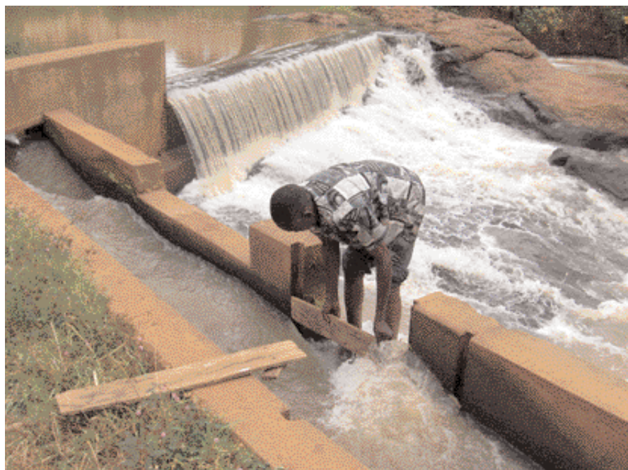
Figure 2: Tungu-Kabiri project – opening spillway
