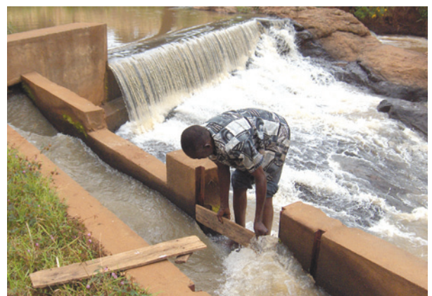
Spillway being opened at the Tungu-Kabiri hydro project in Kenya.
