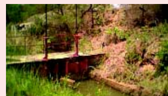
The water inlet in Friedenheim.
