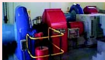
The powerhouse in Friedenheim.
