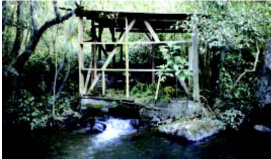
Microhydro installation at a farm near Sabie in South Africa, operating on a head of 84 metres. The turbine is coupled to a 45 kW generator and supplied the whole farm and wood mill. Unfortunately floods in 1999 damaged the plant beyond repair.
